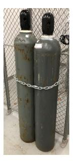
The contents of compressed gas cylinders can pose numerous hazards including but not limited to flammability, toxicity, and asphyxiation. If a space is not properly ventilated or rated for the hazard(s), the atmosphere in a room could become dangerous in the event of a leak. Ideally, spaces storing bulk quantities of compressed or liquified gases should be equipped with air monitoring devices to warn personnel of hazards such as oxygen depletion or explosive atmospheres.
