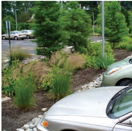
Examples of permeable pavement, pavers, and planted bioretention areas in parking lots
