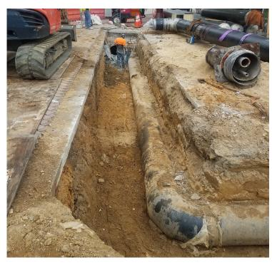
The Glassboro Campus' heating and cooling system includes a substantial network of underground infrastructure that has partially deteriorated and exceeded its useful life. The University has deemed it necessary to replace portions of this infrastructure, which includes chilled water, condensate and steam distribution pipes and the reconstruction or replacement of manholes.
