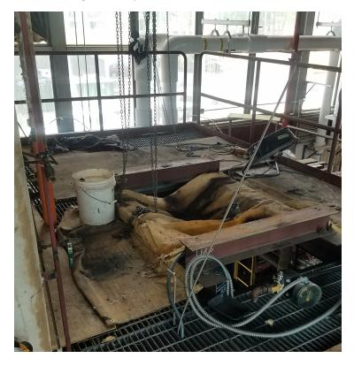
A critical item at the CUP is the underground condensate return tank. Originally built in 1964, this concrete pit has begun to crumble and is being replaced in June with an above ground steel tank, providing more reliability in heating and cooling much of campus. Another important project includes the replacement of boiler tubes in the plant's large co-gen unit, which will extend the life of the unit, and continue to allow the University to create its own electricity.
