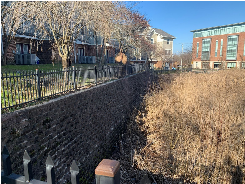
Constructed wetland at Townhouses
