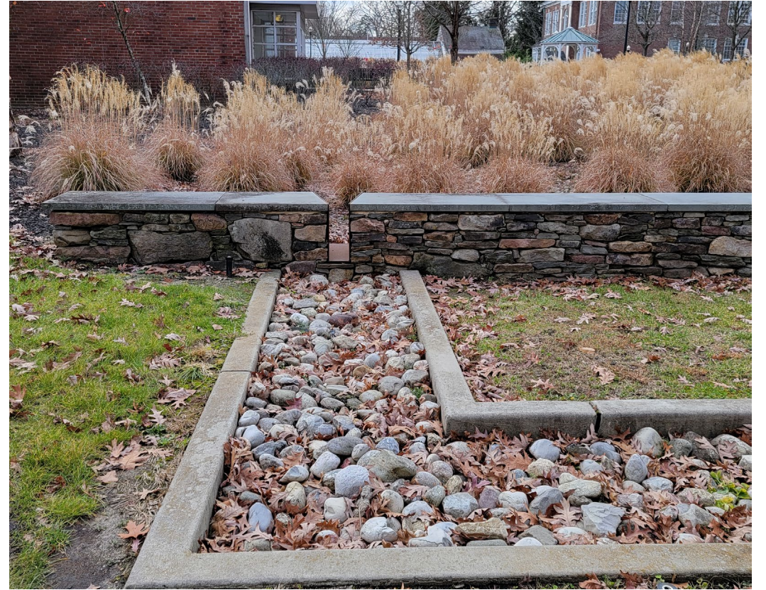
Stone conveyance channel at the Memorial Hall rain garden
