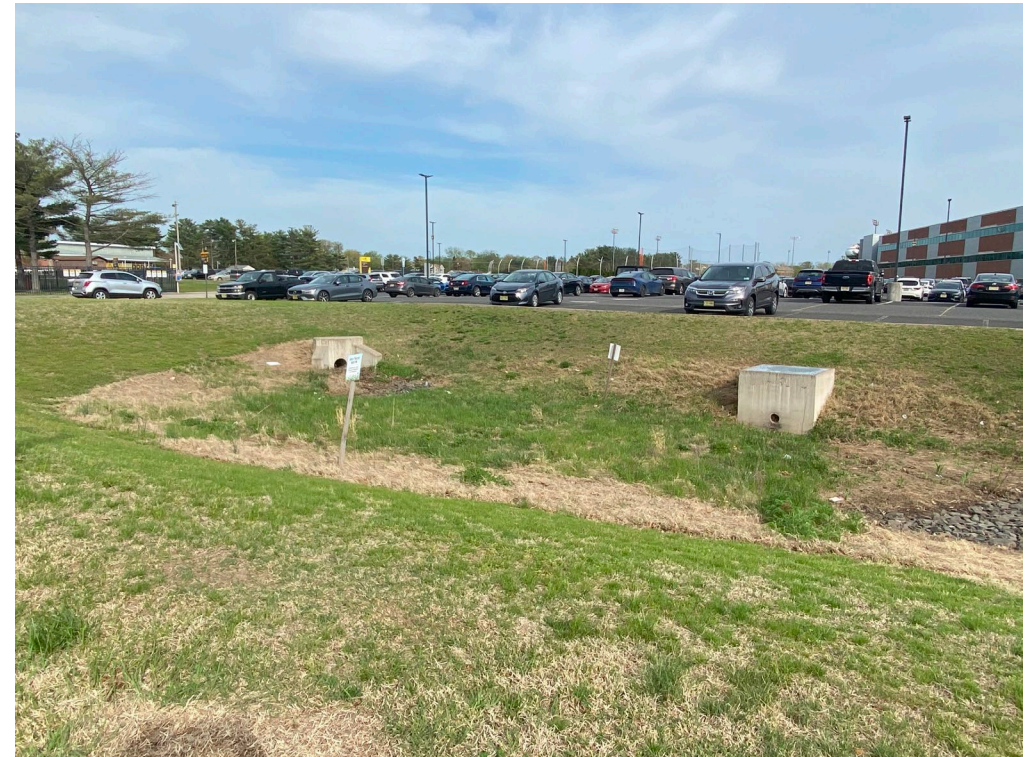
Detention basin adjacent to Lot O
