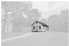
Carpenter Street School, Woodbury, New Jersey 1/15
