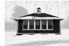
Court Street School, Freehold, New Jersey 2/15
