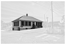
Division Street School, New Albany, Indiana 2/15
